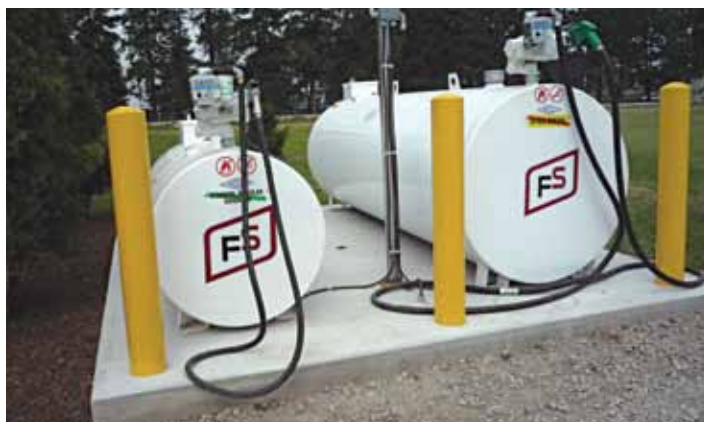
Figure 2.1. On-farm fuel storage with vehicle protection (bollards).
