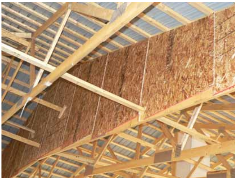
Figure 3.6. Example of an attic fire stop under construction in a new calf barn.
