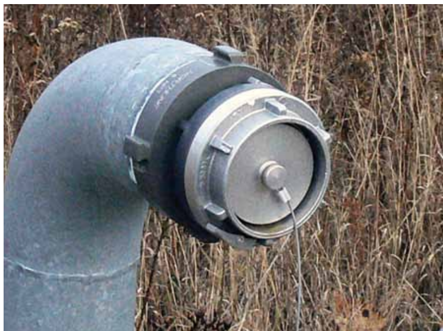
Figure 4.6. Dry hydrant standpipe connection.
