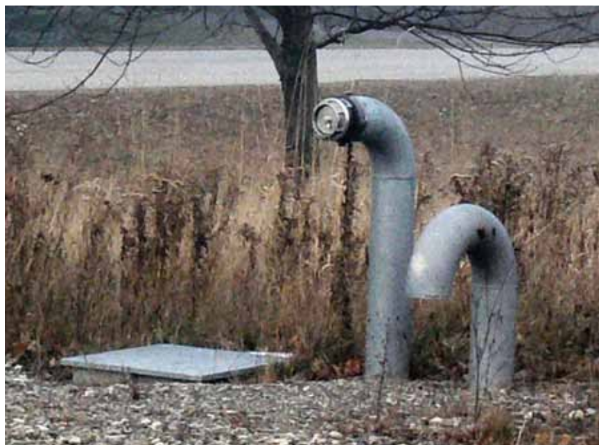
Figure 4.5. Dry hydrant showing all features.
