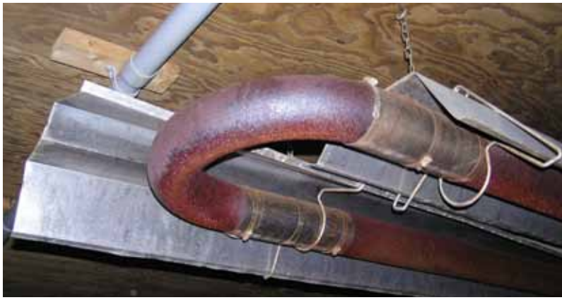
Figure 1.5. Radiant tube heater lacking heat shield. Note close proximity to combustibles (wood ceiling and conduit).
